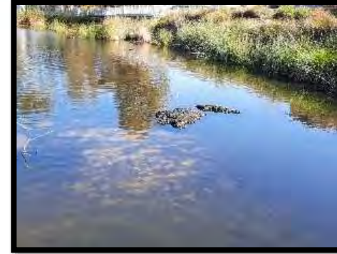
Accumulation of builders sand in Cygnia Cove constructed wetland (after passing through GPT) Photo credit: Perth NRM
