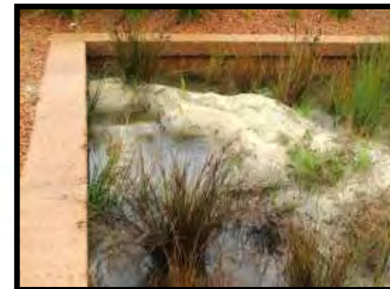
Damaged Sediment Trap, Little Carine Lake Photo credit: Perth NRM
