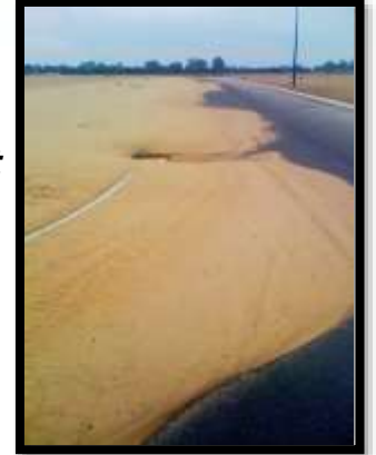
Sand drift and erosion to stormwater entry pit Photo Credit: Swan River Trust
