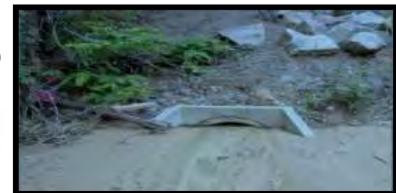
Drain filled with sediment runoff from construction site, Kenwick Photo credit: Perth NRM
