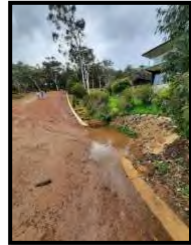
Drain filled with sediment runoff from construction site, Kenwick Photo credit: Perth NRM
