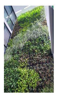
A green wall is a vertical structure planted with vegetation that contains a growing medium and a built-in irrigation system.
