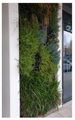
Other considerations for green wall design include the load-bearing capacity of the location and access for installation and maintenance. Regular, scheduled maintenance is a critical success factor for healthy green walls. This includes fertilisation of the plants and Deep Green recommends application via the reticulation system to provide appropriate nutrients directly into the plants root zone.
