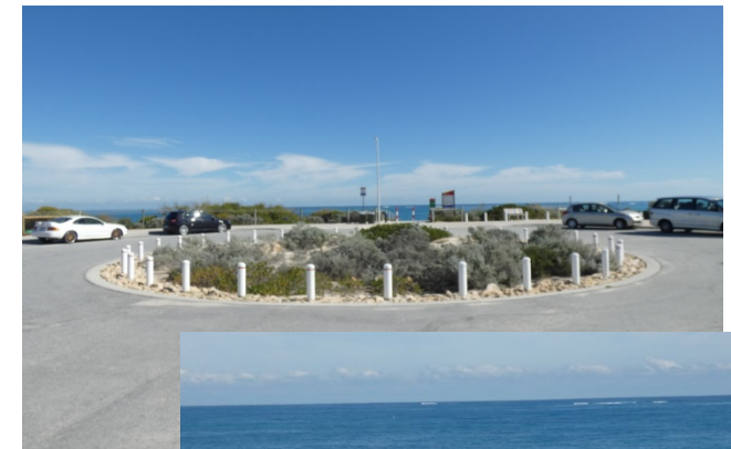
Images: Stormwater from car parks directed into vegetated areas to manage flows and pollutants
