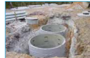
Stormwater pits
