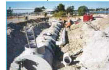
Stormwater pits
