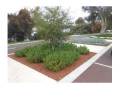
Where roadside car bays are incorporated into the verge, the biofilter beds are interspersed with poured limestone paths to allow pedestrian access to the footpath without disturbing the vegetation.
