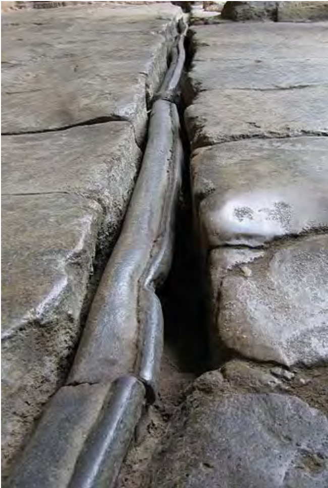
Lead water pipes
