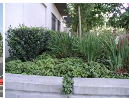
Building Bioretention Planters (Portland, Oregon, USA)
