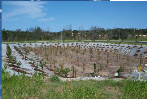
Bracken Ridge Bioretention Basin (BCC)
