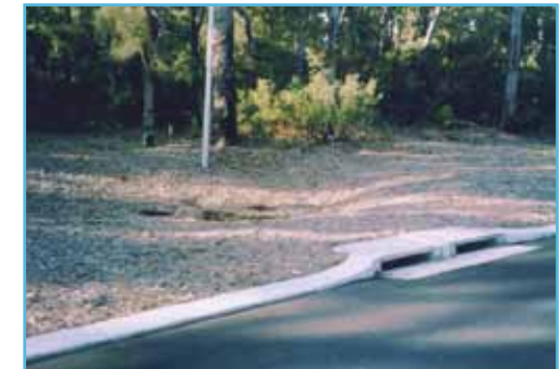
Completion, Boronia Ridge, Walpole
