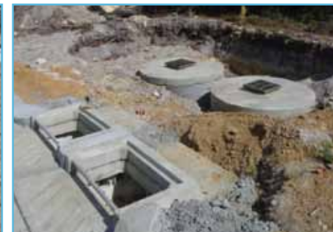
Installation, Boronia Ridge, Walpole
