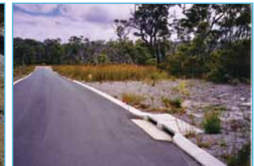
Completion, Boronia Ridge, Walpole
