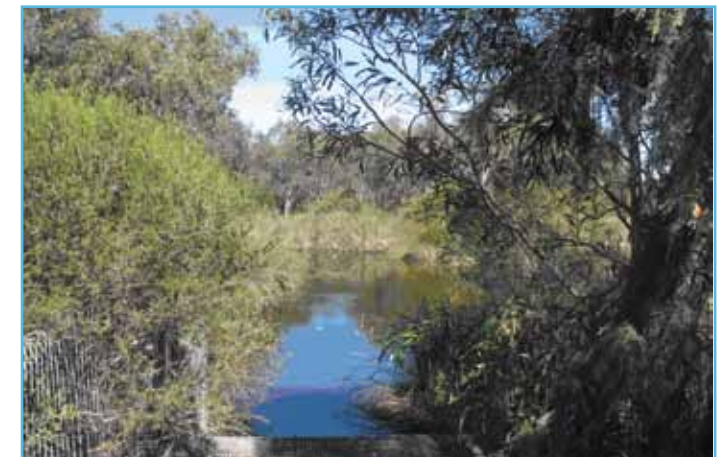
Lieve Street constructed wetland, Cannington
