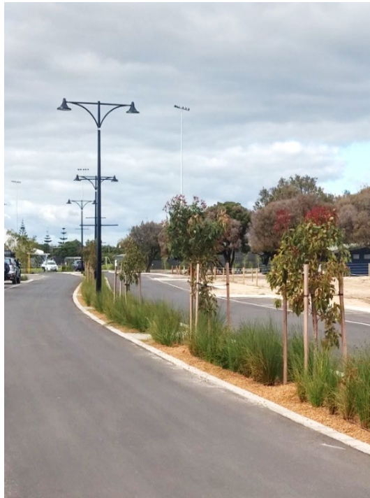
Figure 3: Roadside swale for treatment of stormwater
