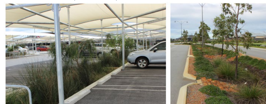
Figure 2: Car park biofilter and roadside swale
