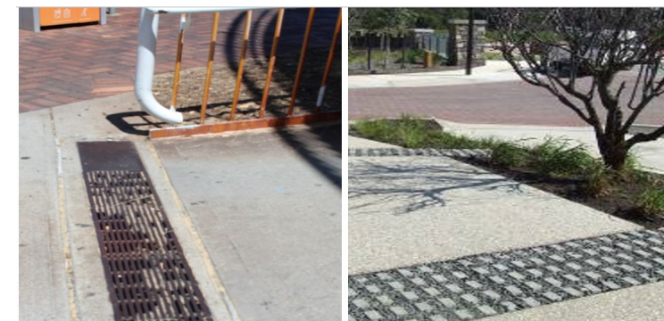
Figure 5: Disconnecting hard surfaces (grates and permeable pavement) reduces stormwater flows
