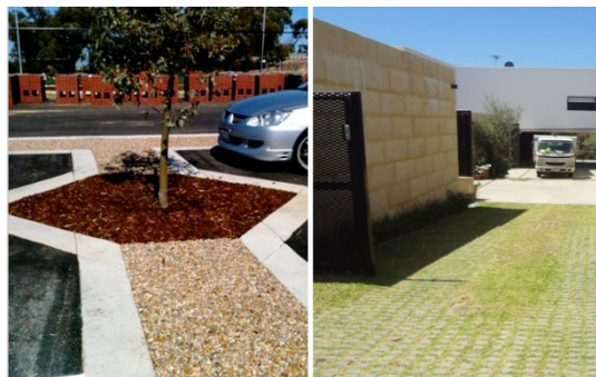
Figure 4: Permeable pavement types
