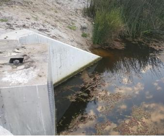
Outflow pipe and floodgate Overflow weir - high tide
