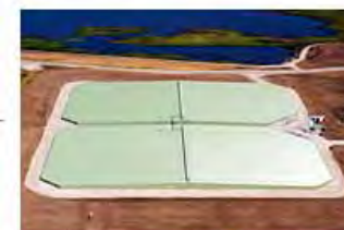
Chlorine contact basins
