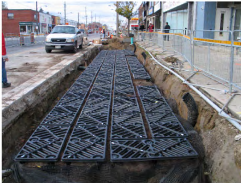
Silva Cell decks go on
