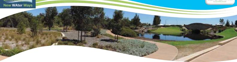
The Siroi Court site comprises multiple WSUD best practices. This includes the innovative use of a constructed treatment lake for the storage and treatment of shallow groundwater for public open space (POS) irrigation, a biofiltration basin to treat stormwater runoff generated from adjacent roads during small events, and a revegetated buffer zone to rehabilitate adjacent conservation category wetland, Balannup Lake.
