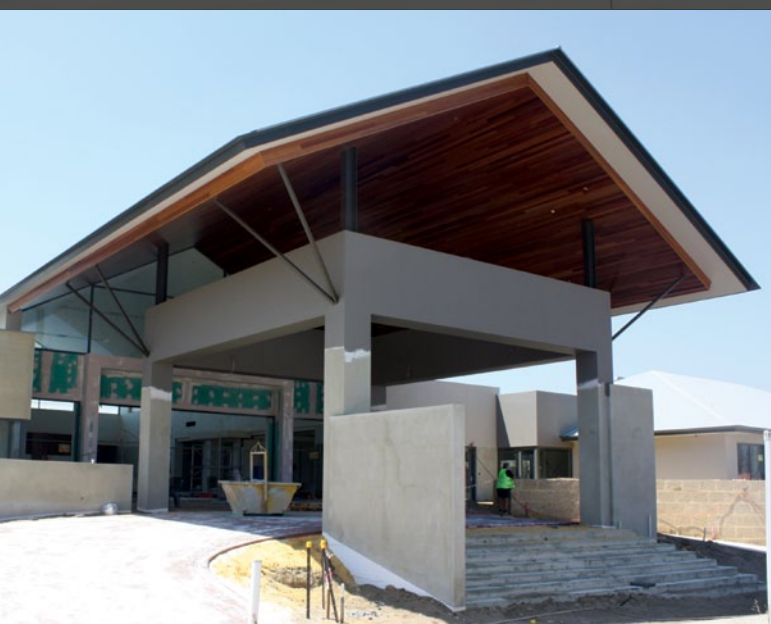
Dramatic entrance canopies such as this enhance the visual amenity of the area and provide effective solar shading
