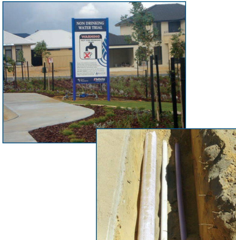
The use of a purple-pipe system to supply an alternative fit-for-purpose water source for irrigation (courtesy of the Satterley Property Group)
